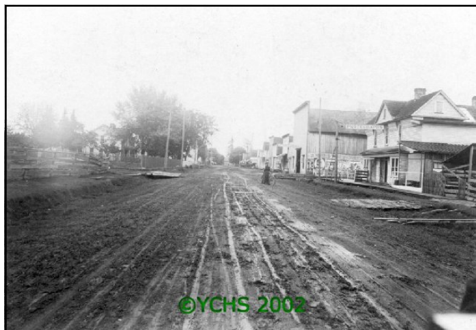
Amity Trade Street Looking Southwest
