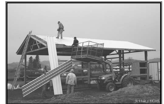
Volunteers installed the sawmill roof.
